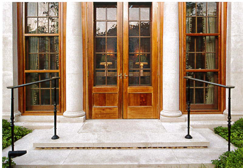
The custom triple-hung windows and glass-filled doors allow in a lot of natural light, blending the vision of indoors and outdoors. The restoration glass speaks of the past.
