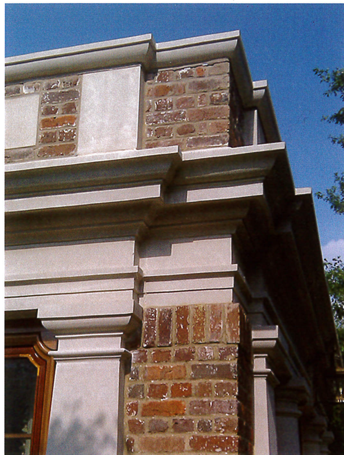
Internal downspouts at the corners of the folly wash the water to the ground, giving the illusion that the single-room building is a thing of the distant past.
