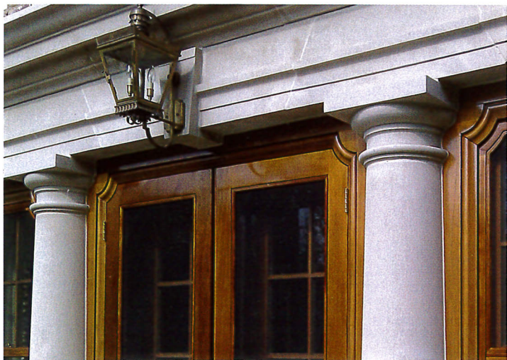
The curves of the custom Spanish cedar doors and frames echo those of the Indiana limestone capitals.
